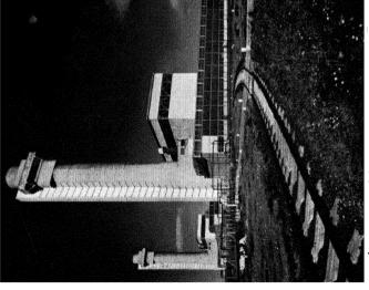
6. The two giant reactors of the Windscale atomic explosives factory. The long low building is one of the four halls housing fans used to cool the reactors. Resultant hot air is expelled through the 410-ft-high chimneys. Service lifts run in the oblong-shaped tubes to the left of each chimney.
