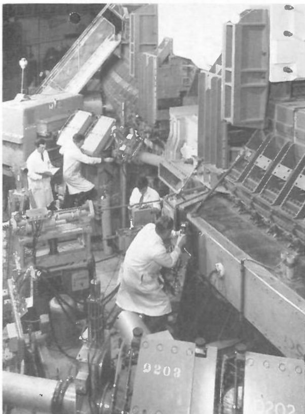
Fig. 3 April 1964. Final checks on the high energy beam lines emerging from Nimrod.
