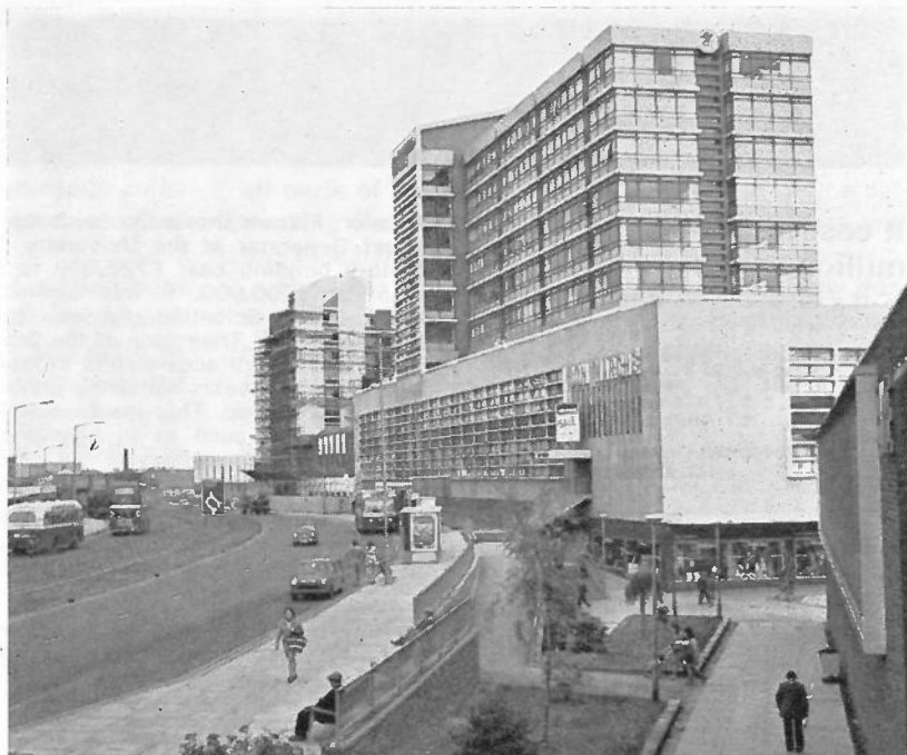
New offices, shops and a large hotel (l) in Fleming Way, Swindon. The Parade shopping centre lies behind them Published by courtesy of Swindon Corporation
