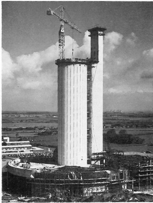
Picture shows progress made on the Nuclear Structure Facility (NSF)
