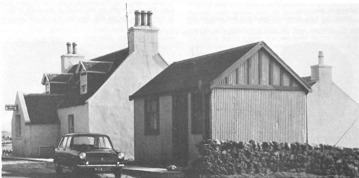
The Ben Mor Guest House, South Uist, with the annexe in foreground of picture.
