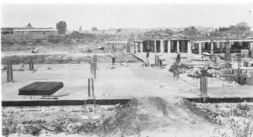
Swindon office starts to take shape
