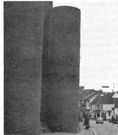
The outside of the new shopping centre dwarfs old Basingstoke.
