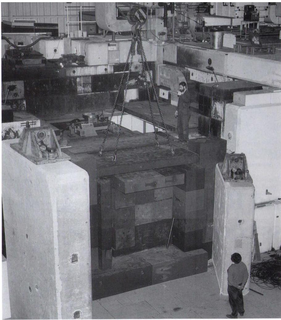
Figure 1: Modifications to the extracted proton beam at Isis showing the steel shielding for the RIKEN pion injection system.
