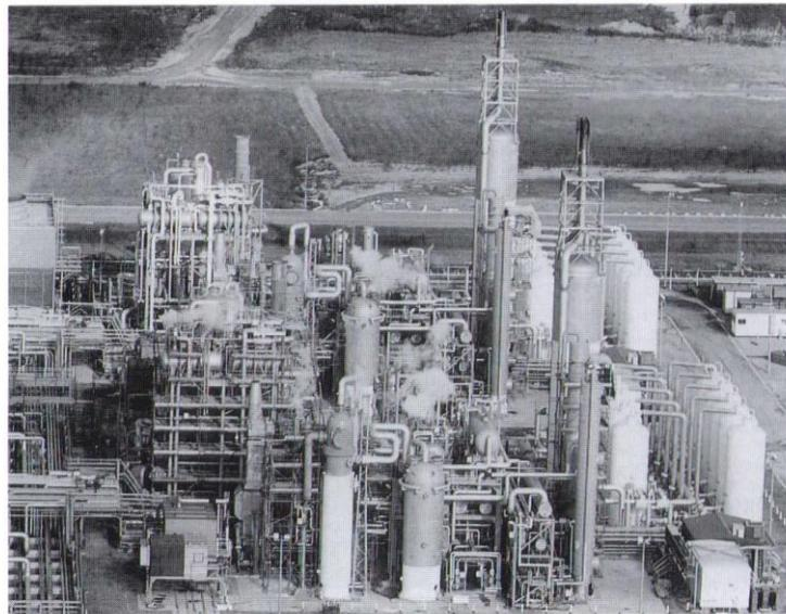
The new leading concept ammonia technology for ammonia production developed by ICI virtually eliminates sulphur dioxide emissions and reduces nitrous oxide emissions by a factor of seven compared with previous technology.
