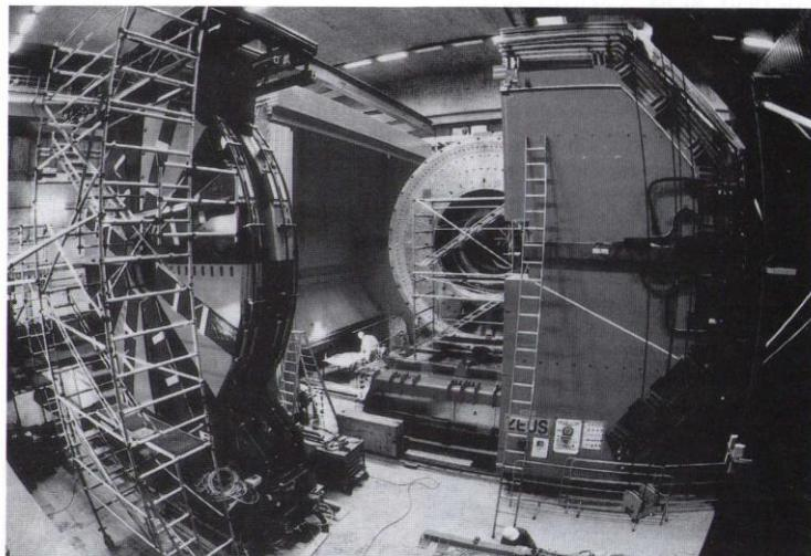
A view of the ZEUS experiment during the installation of the components. The picture was taken before the installation of the tracking detector built by the UK groups in ZEUS. This detector fills the central cylinder seen in the picture.
