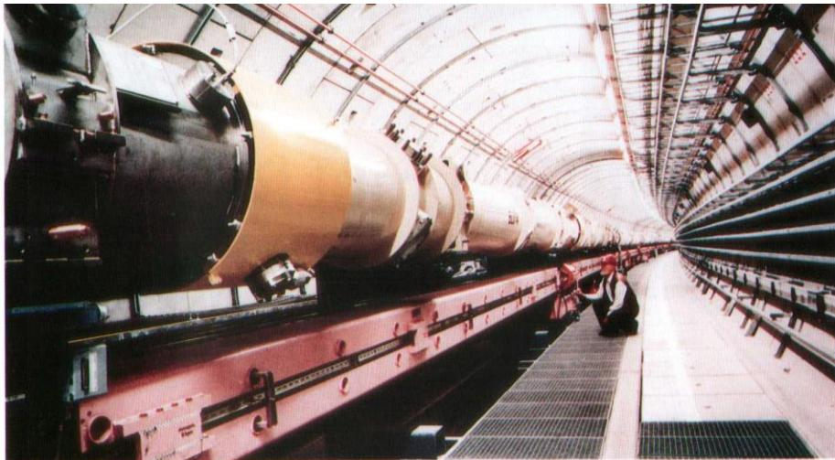
A view of the HERA tunnel in which electrons and protons are accelerated to very nearly the velocity of light. The four-mile tunnel runs under the outskirts of Hamburg in Germany. The protons and electrons each travel in their own evacuated pipe, and are guided round by magnets. The large cylinders are the cold superconducting magnets which guide the protons and underneath are the smaller "warm" magnets which guide the electrons.
