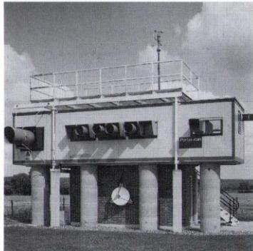
Figure 3: The transmitter cabin at Chilbolton. Equipment is mounted on benches supported independently from the cabin, on steel pillars within the concrete tubes.
