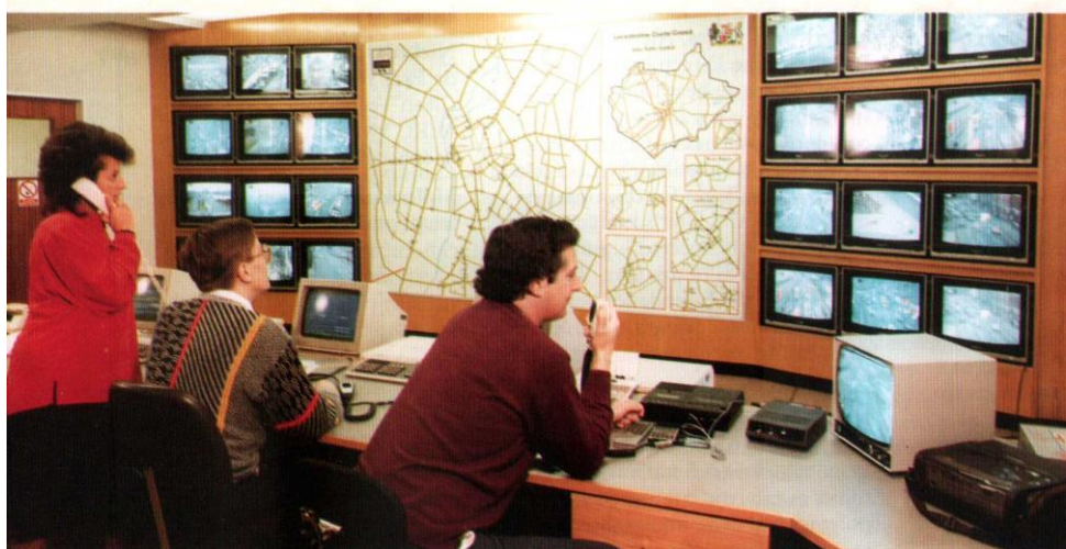
Traffic operators at Leicestershire County Council, by adjusting the traffic signal timings, alleviate congestion observed on closed circuit television. Research funded by SERC at Nottingham University Transport Research Group is investigating the effect of congestion control on air pollution and noise levels. The feasibility of automatic remote monitoring of the environment integrated with traffic monitoring is being investigated in collaboration with Siemens Plessey.
