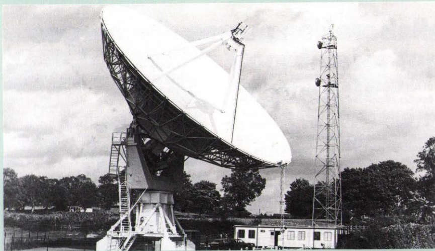
The 25m E-Systems dish at Knockin. The L-Band and Microwave Link communications dishes are on the tower adjacent to the building.
