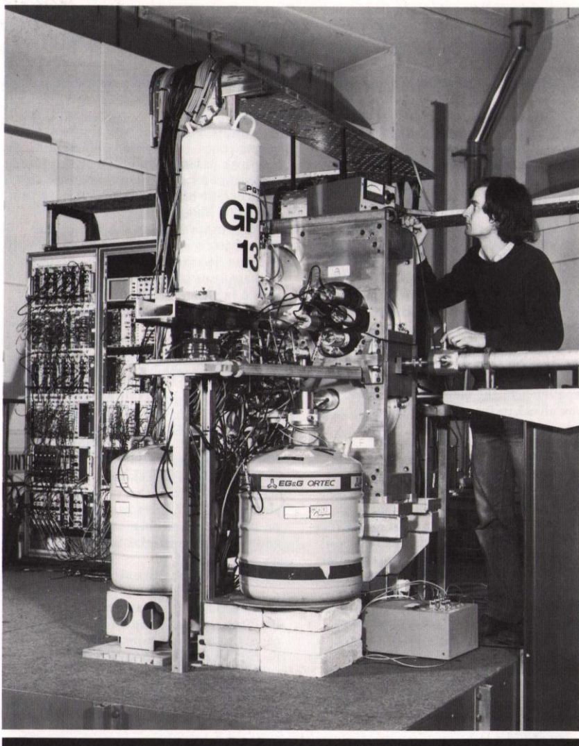
The experimental equipment TESSA II showing the liquid-nitrogen cooled detectors and associated equipment surrounding the target location used in the studies of rapidly rotating nuclei.
