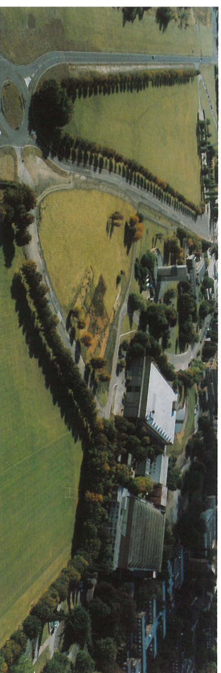
Aerial view of Harwell showing redevelopment area at the left. (UKAEA 1700)
