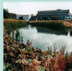
The Hangar 9 lagoon balances rainwater surges on site.
