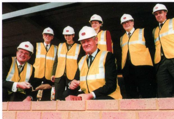
Laying the foundations for new development at the Harwell International Business Centre, UKAEA chairman, Sir Kenneth Eaton (right) and John Cutts, chief executive, ProLogis.
