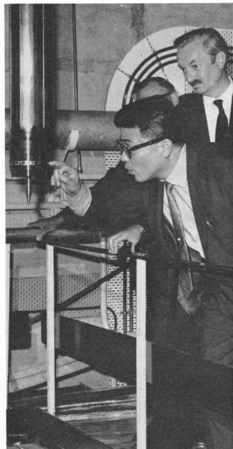
IRRADIATION SERVICES. A fuel element for the Japanese heavy-water reactor (FUGEN) is inspected prior to irradiation in the Winfrith SGHWR.
