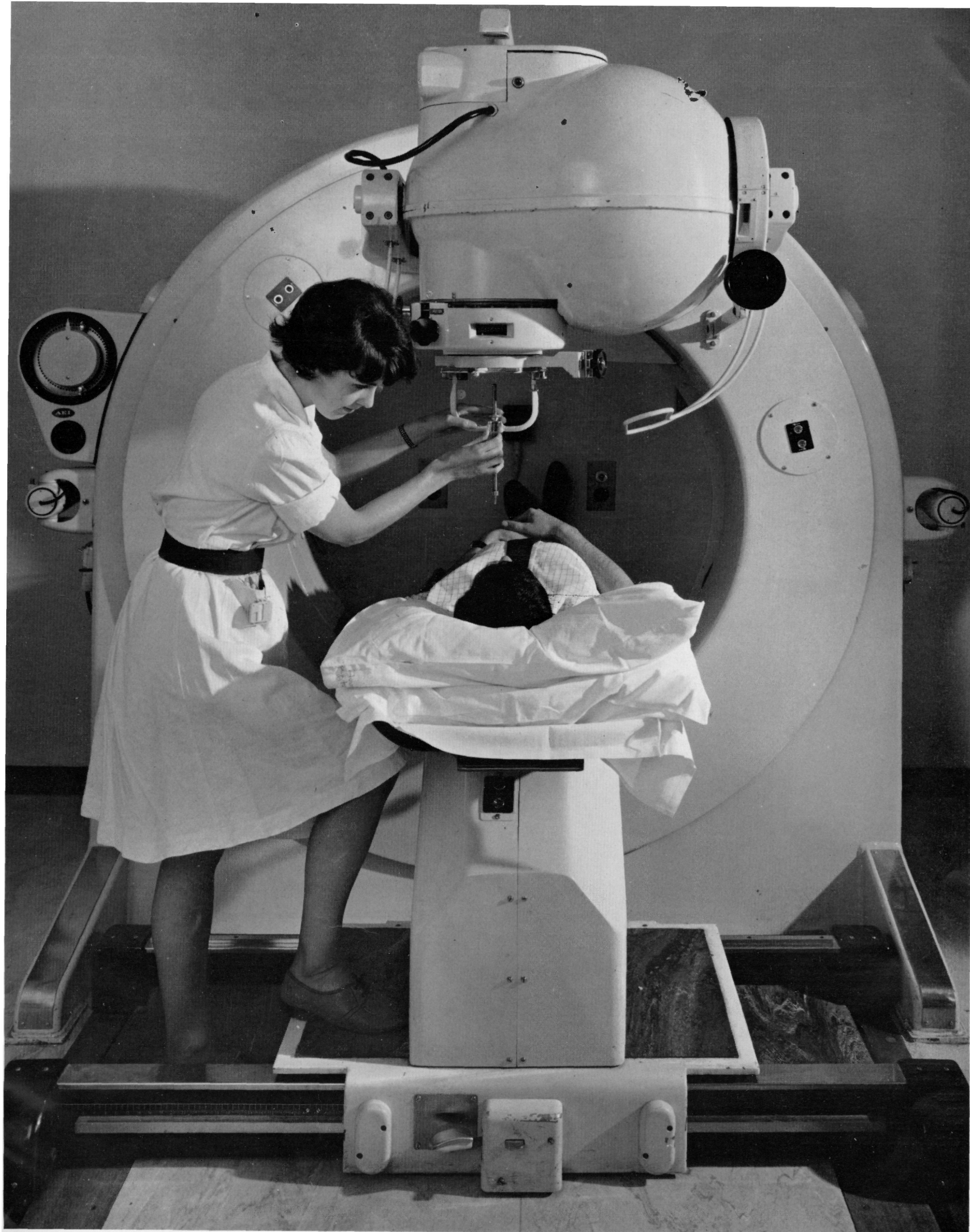
THE ISOTOPE PRODUCTION UNIT at Harwell supplies Cobalt 60 for use in radiotherapy. At St. Luke's Hospital, Guildford, the patient is positioned under the 5000 Curie Cobalt Unit, which then rotates round him, directing the radiation to the exact point requiring treatment.
