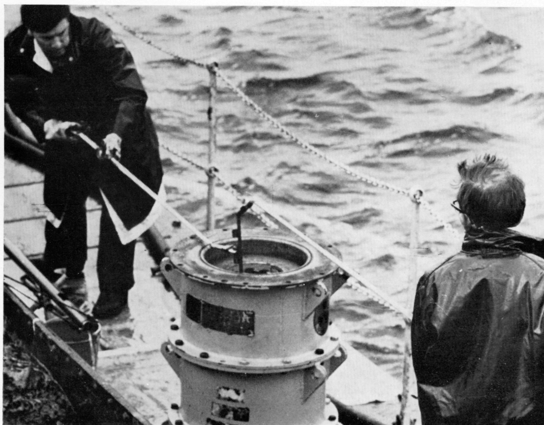
SILT MOVEMENT There has been a considerable expansion of the use of radioactive "tracers" for the study of the movement of silt in estuaries. An investigation in Swansea Bay established the suitability of a site for material from the new iron ore terminal at Port Talbot. Two others in the Severn Estuary confirmed the acceptable dispersal of material dredged from Newport and deposited in Newport Deep. A study of silt movement in the Clyde Estuary is being conducted in collaboration with the University of Strathclyde.
