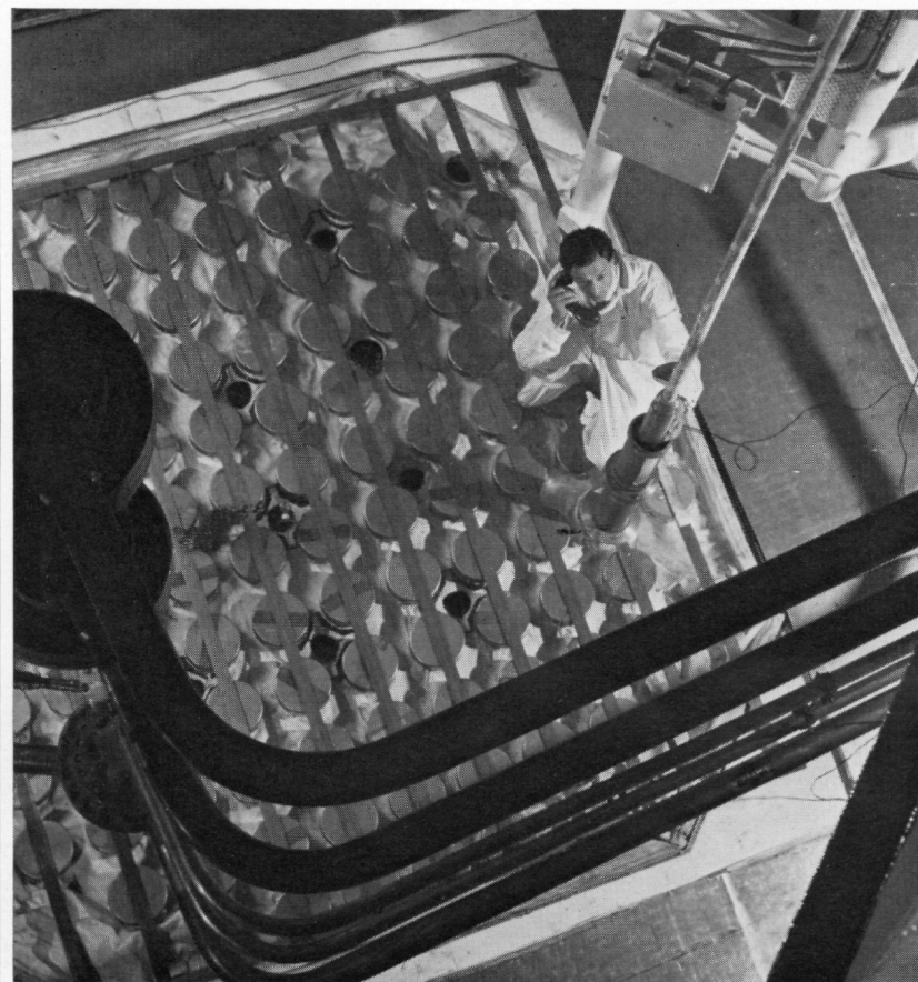
S.G.H.W.R. A view of the charge-face of the Steam Generating Heavy Water Reactor at Winfrith which is programmed to go on power at the end of 1967. Shop-fabrication of all major reactor components allows a comparatively short construction time on site.
