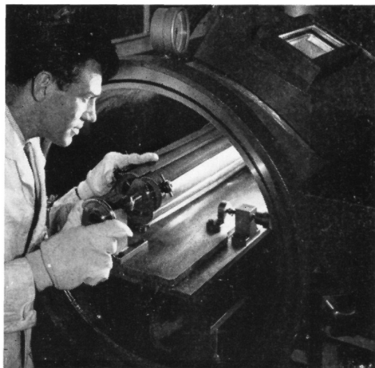
Fuel element plates for materials testing reactors in Britain, Australia, Denmark and Germany are manufactured at Dounreay.
