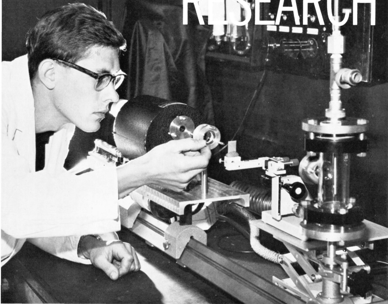
Adjusting high-energy laser equipment at Harwell prior to a can-puncture experiment. Fuel cans are punctured inside a vacuum apparatus so that the fission gas can be analysed.
