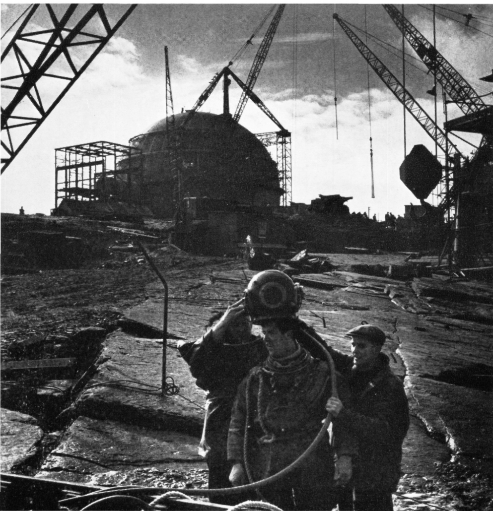
The fast breeder reactor at Dounreay had reached this stage in March, 1957. The diver in the foreground is about to undertake drilling operations in the rock of the sea-bed.
