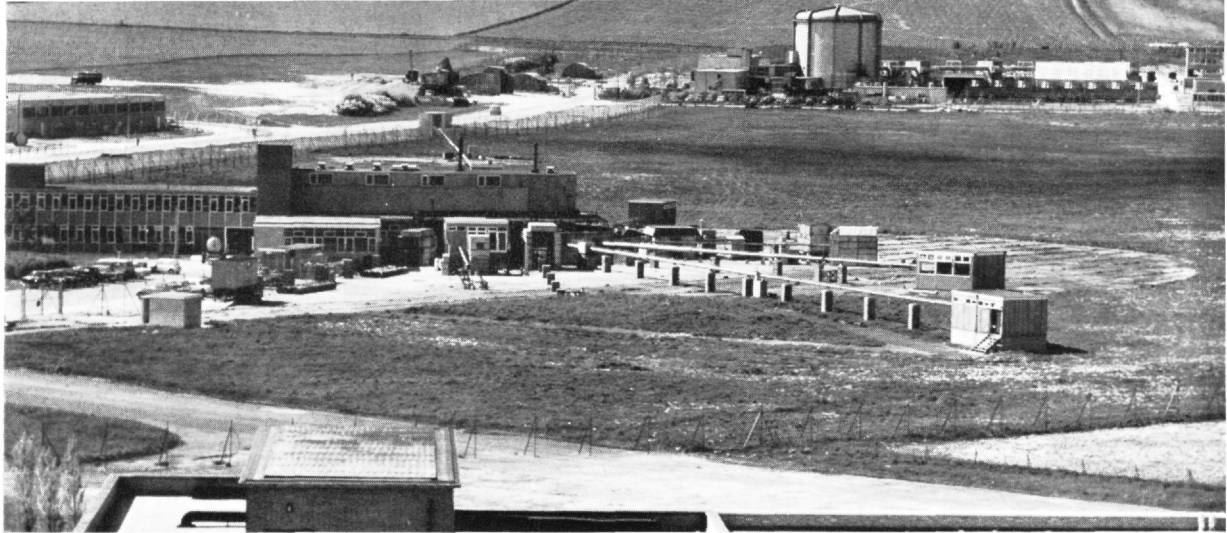
The neutron project at Harwell. In the right foreground are the flight tubes radiating from the target room.
