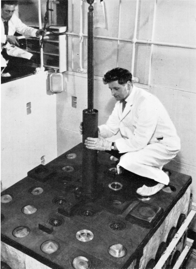
FIFI (Fine Flux Investigations Facility) is used at Windscale to study fuel for A.G.R. and other reactors.
