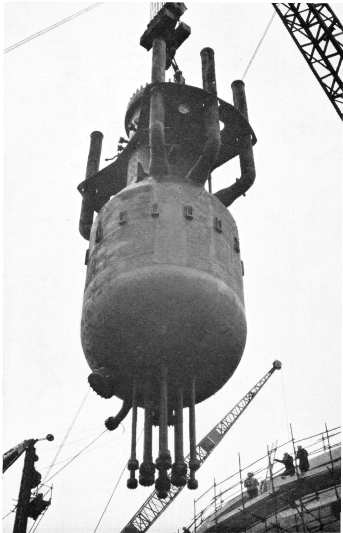
The 48-ton pressure vessel being loaded into the DRAGON high temperature reactor at Winfrith.
