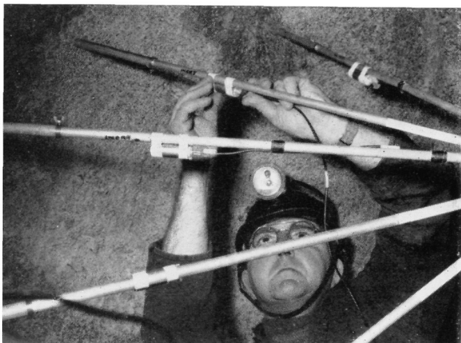
To study methods of detecting nuclear explosions, the Weapons Group fired conventional explosives underground. Picture shows preparation of a charge at Kit Hill Mine, Cornwall.
