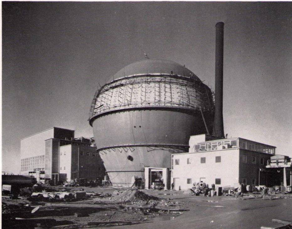
ADVANCED GAS-COOLED REACTOR. A general view (February, 1961) of the experimental A.G.R., now nearing completion at Windscale. It is planned to begin operation towards the end of 1961. The main objective of the A.G.R. is to reduce the capital cost of the reactor installation.
