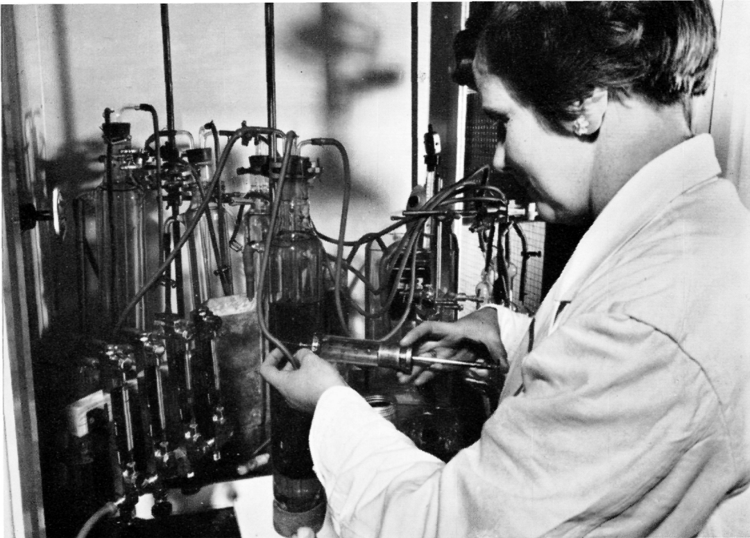
Producing a radioactive form of one of the B vitamins at the Radiochemical Centre, Amersham.
