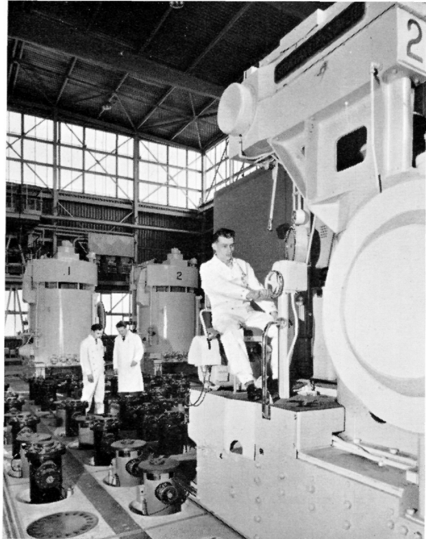
Loading fuel elements into No. 1 reactor, Chapelcross.
