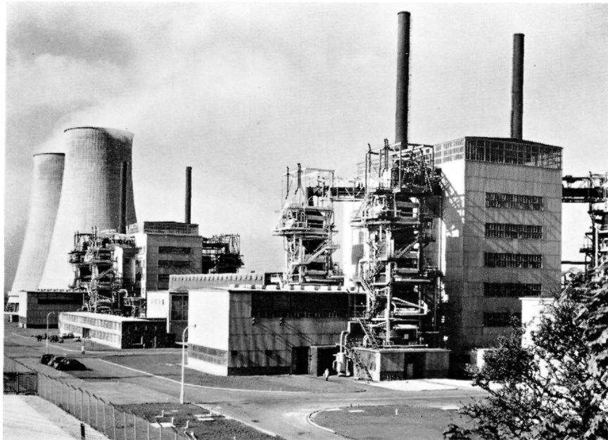
CALDER HALL, CUMBERLAND. Four reactors - 184 MW. Officially opened 1956. Dual-purpose station for plutonium production and electricity generation.
