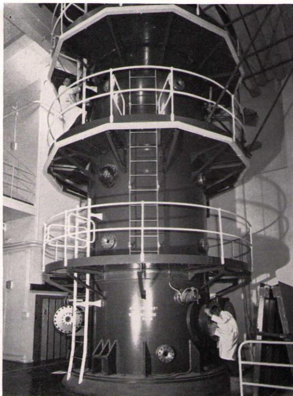
TANDEM ELECTROSTATIC GENERATOR, ALDERMASTON. This machine and a similar accelerator at Harwell are designed to yield basic information on the behaviour of nuclei which will be of value over a wide range of the Authority's research and development programmes.
