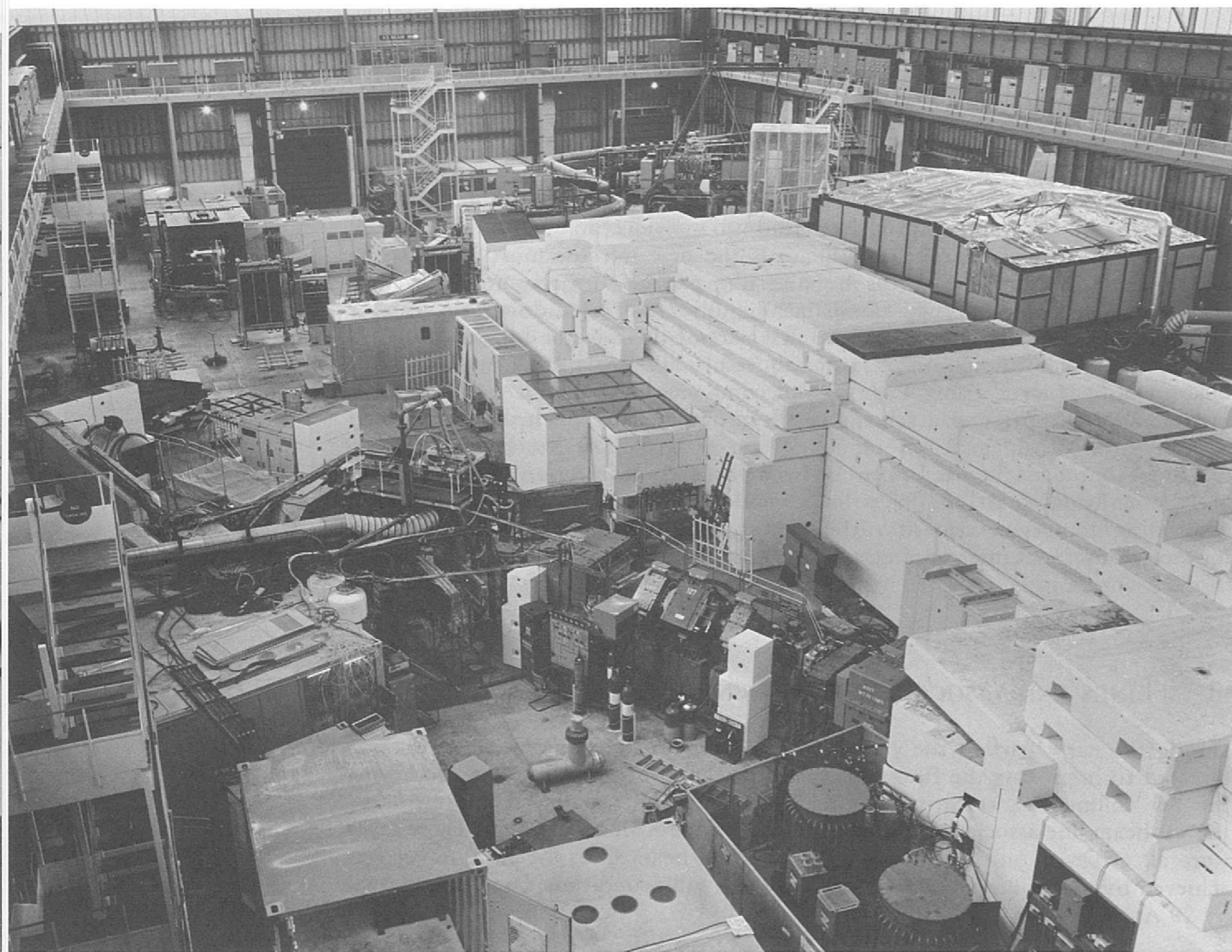
Figure 95. General view of the Experimental Hall 3 showing the K15 beam line and the X3X blockhouse.
