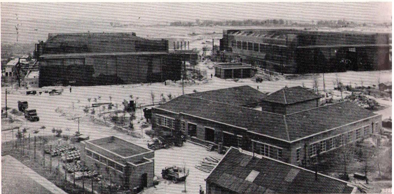
A corner of the Chilton pre-fab site is just visible in the top right-hand corner of this photograph. The houses were built so that one of the old airfield run ways provided the road between them. Beside such signs as "Danger: do not move doors", contractors' lorries and Post Office telephone engineers were busy around hangars which still had their wartime camouflage paint.
