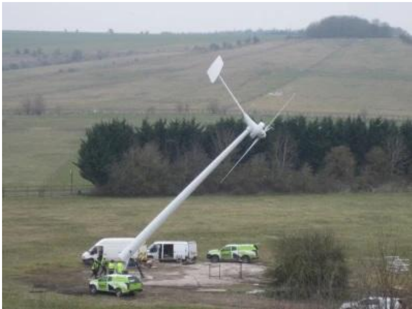
Installing the new wind turbine in February 2018.
