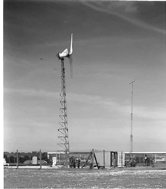
North Wind Turbine in 1986.
