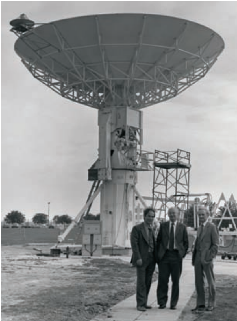
The newly formed Rutherford Appleton Laboratory's Director General Dr Godfrey Stafford, together with Dr Geoff Manning, Director, Rutherford (left) and Dr John Houghton, Director, Appleton (right) stand in front of the new IRAS dish. IRAS, a 12 m diameter, fully steerable S-Band antenna from NASA, was constructed at RAL in 1979. It also acquired a complete unified S-band telemetry and command system, which had originally served the Apollo missions at the Madrid tracking station.
