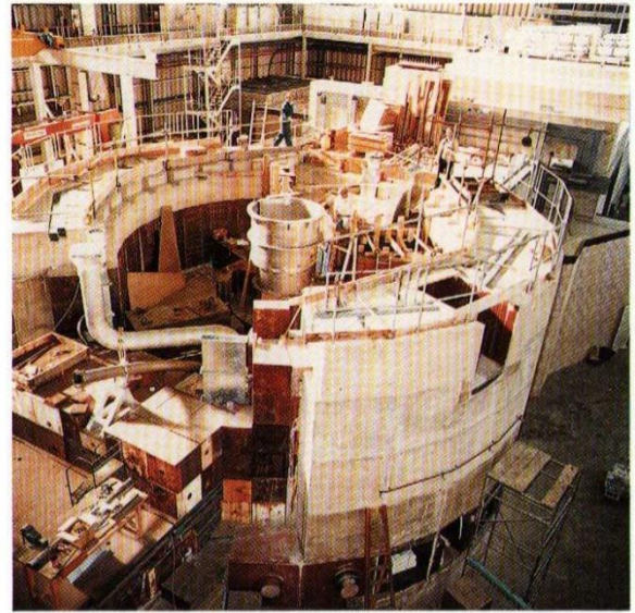
ISIS target station under construction.
