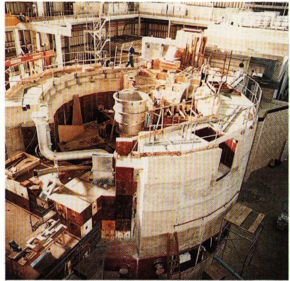
The ISIS target station under construction.
