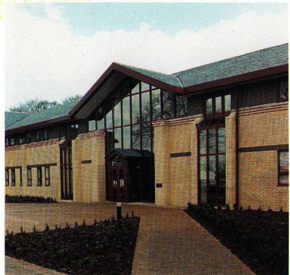
The SERC's new Royal Greenwich Observatory building in Cambridge - designed and constructed by the Council Works Unit.
