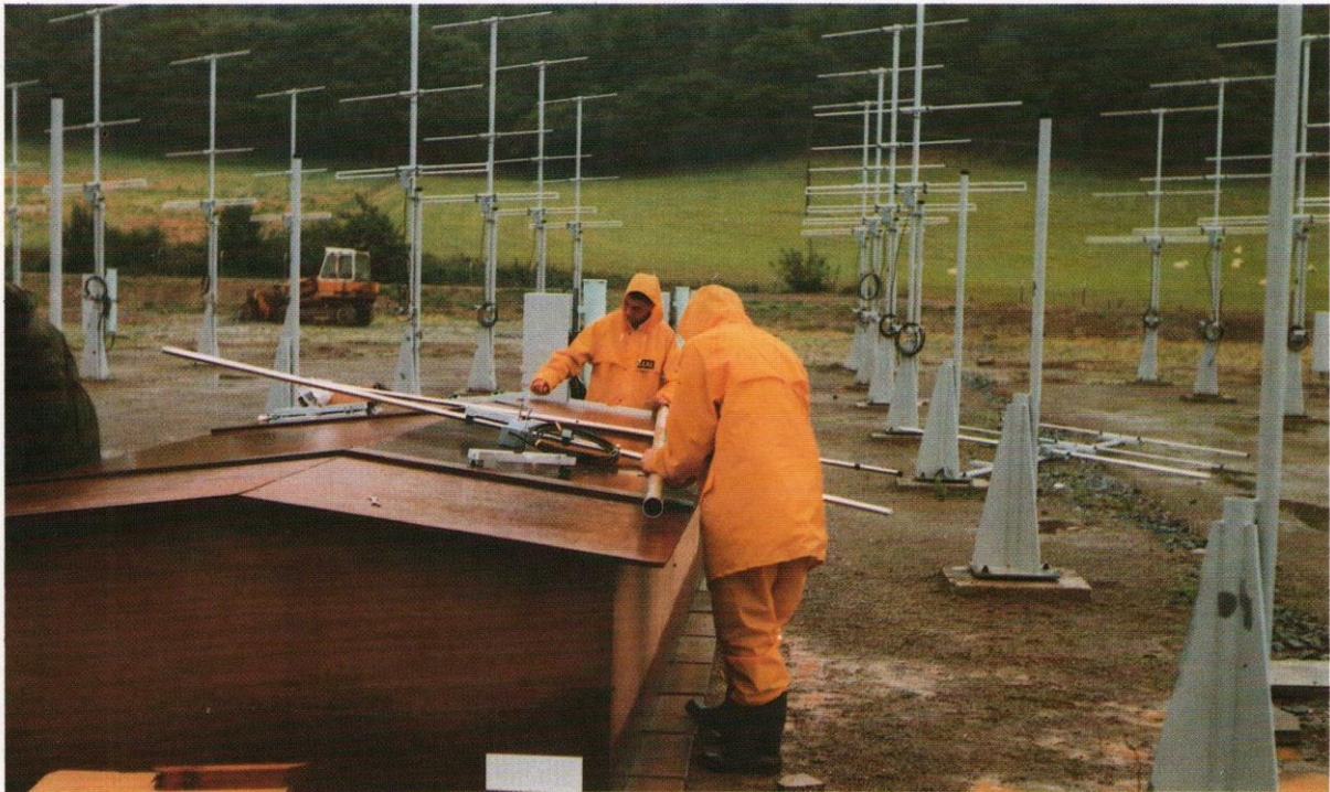
1.11 MST radar array at Aberystwyth.
