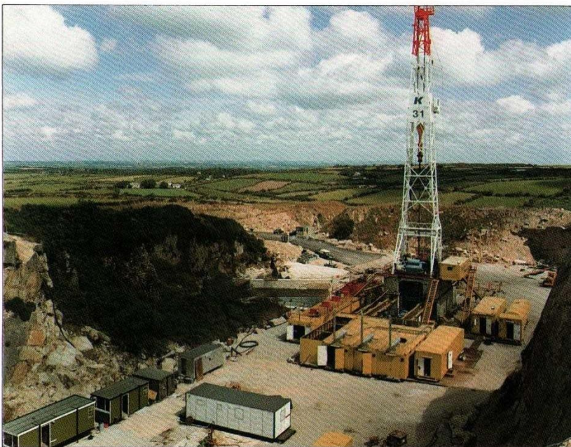
Geothermal Energy Research at Rosemanowes Quarry, Cornwall. (Camborne School of Mines).
