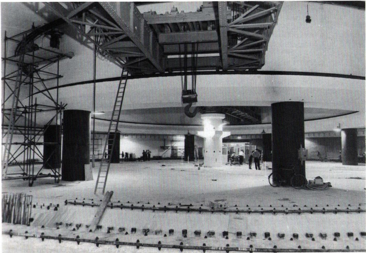
Fig 15. Inside the magnet room. Floor datum points were used to accurately survey the location of the sectors and pole pieces.
