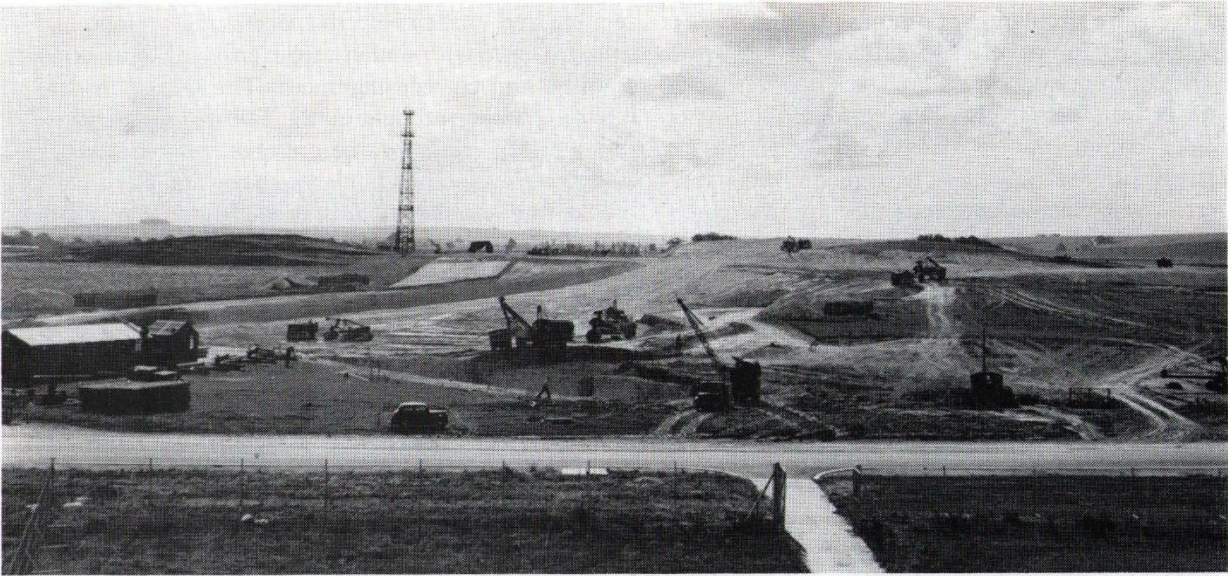
Opening up the site.
