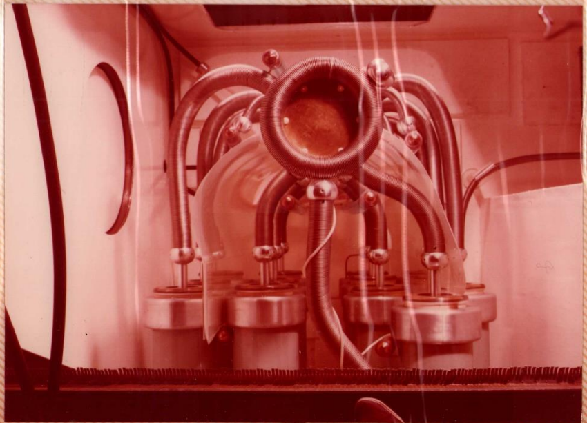
PLATE 24 (NEG. 27811) Top view of output end of Marx bank showing connecting tubes between capacitors and spark-gap column.
