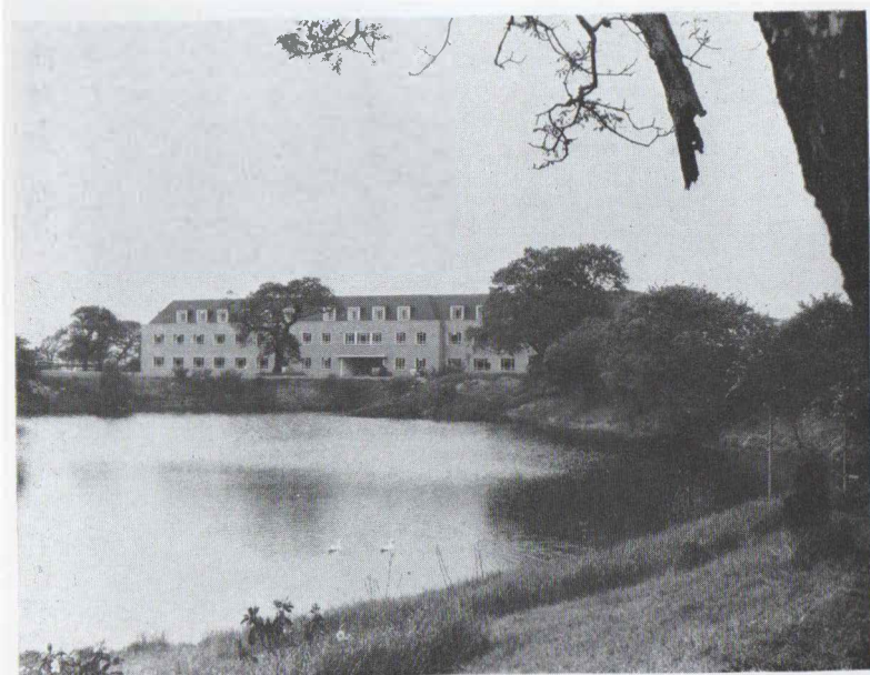
A general view of the works administrative building at Capenhurst
